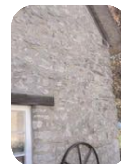
Inappropriate hard cement mortar
